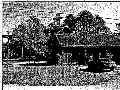
Hilliard Community Center
